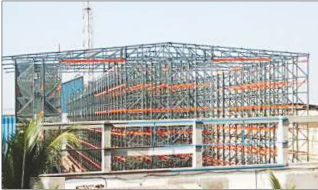
RSW (Under Installation)
