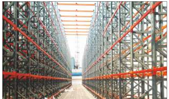
RSW (Under Installation)
