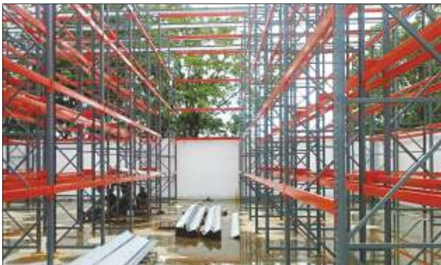
RSW (Under Installation)
